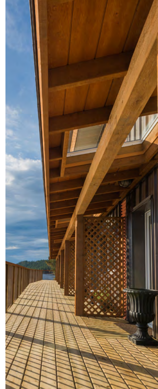
Photo: Bella Bella Passive House provides staff housing for employees at the ł'uxváłásu'ílas Heiltsuk Hospital in Bella Bella, BC. The prefab structure includes six, two-story attached townhomes.
